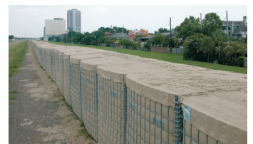
Levee upgrade, East Jefferson, Louisiana
