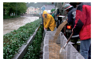
Hesco flood barrier control, Austria
